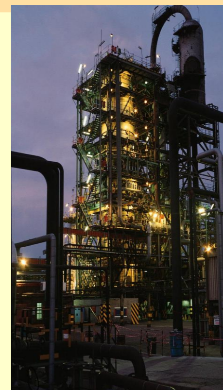
Slurry reactor for Fischer-Tropsch synthesis Source: www.sasol.com
