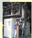
Catalytic pyrolysis pilot unit, CPERI, Greece
